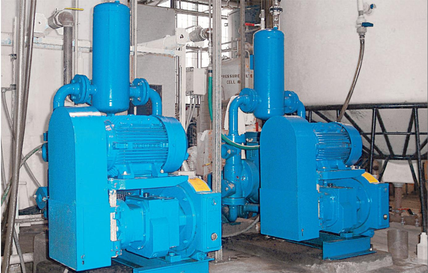
ABEL HMD-G-12-0060 for transfer of contaminated sludge from soil washing process
