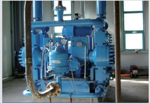
ABEL HMQ with reverse valves for transfer of fly ash with portions of coarse bottom ash
