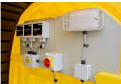
Where a mixer is in use for maintaining the suspension of lime chemical, the power is drawn from the dosing unit.
