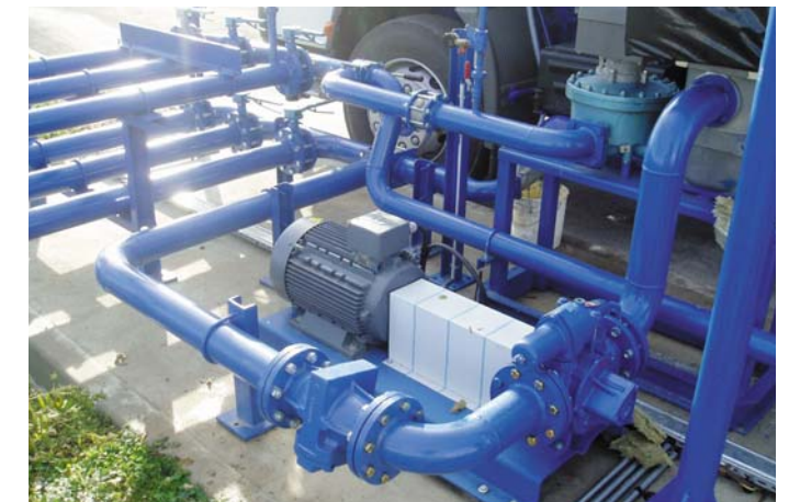
Truck unloading (Diesel)
