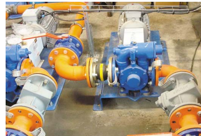
Heating Oil transfer
