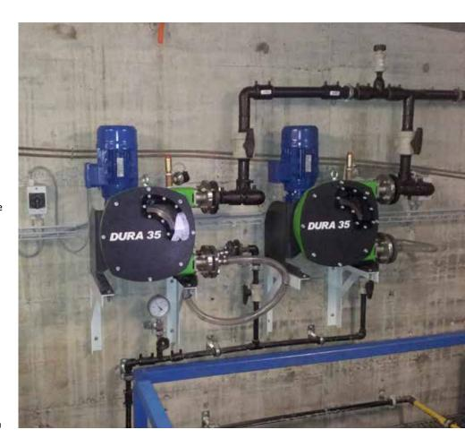
consists of a hose, which is housed in a casing and squeezed by a rotor. As the only part in contact with the fluid is a flexible hose, the pump can run dry and certainly tolerate air in the pipes. The pump itself was sized to run slowly, so as to increase the hose life. The estimated running time of less than 1200 hours per year with
