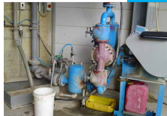
the replaced Abel pump
