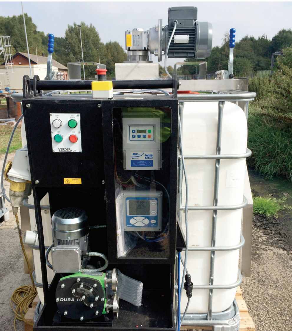
A Verder dosing system delivering Neutralac®SLS45 liquid lime. Here, the dosing rig has been forklifted into position on pallet.
