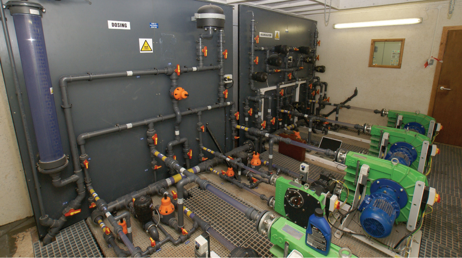
Operational Verderflex peristaltic pumps on a skid mounting, delivering lime. The system was designed, built and installed by the Verder Service Team.
