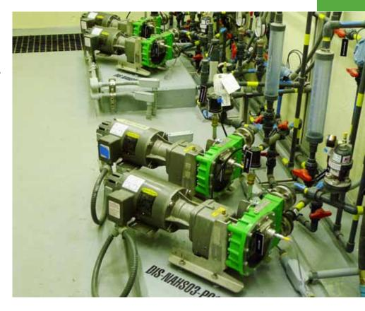
liquid. This process is knows as peristalsis and is what makes the peristaltic pump the first choice for liquid metering. Variations in hose type allow for low strength and even high strength hypo dosing.
