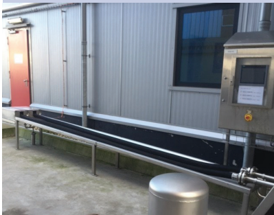
Suction connection tank - pump
