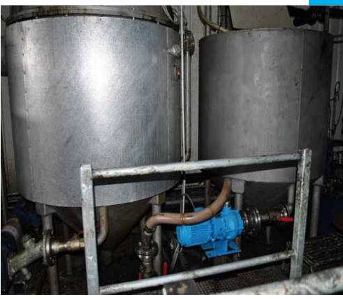
The pump was praised for its ability to handle abrasive media and the multitude of debris that had entered the process from the diverse range of food product that had been delivered to the site including broken ceramic and metal particles. The Verderhus has been installed without incident for several months, outlasting the rotary lobe pump, which had not lasted for more than 2 weeks without failing.
