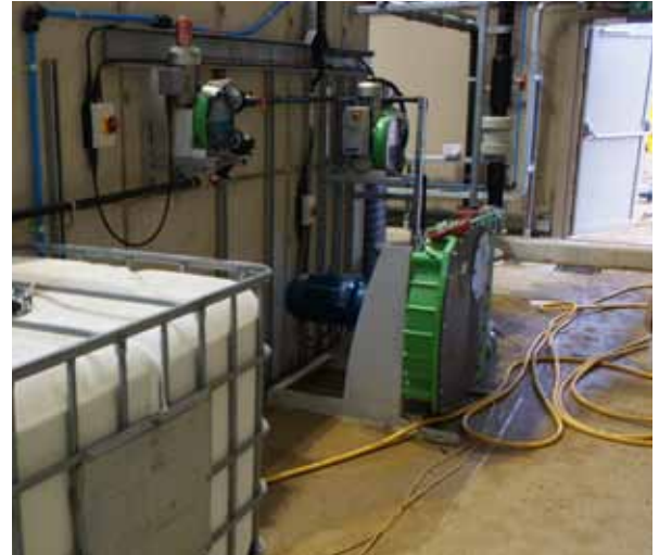
dosing a pH buffer into organic matter
