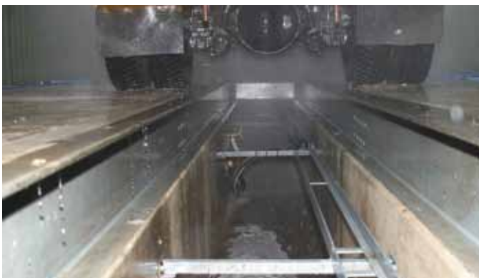
Pumping dirty and recycled water at a commercial car wash is an everyday function for Hydra-Cell pumps.
