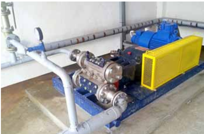
Hydra-Cell T100 pumping gasoline in a distribution centre.
