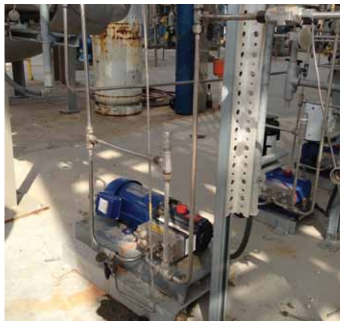
Hydra-Cell pumping ethanol-based liquid for making jet fuel.
