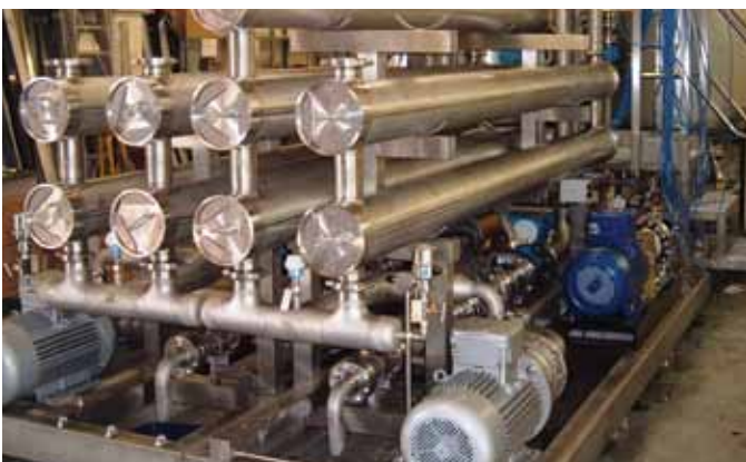
Pumping for waste stream reduction and salt solution concentration at a pharmaceutical chemical plant
