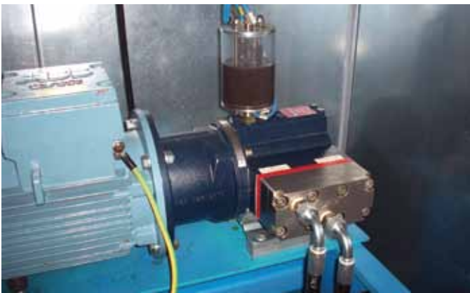
High-precision dosing of pentane at low flow rates can be achieved for specialised applications in polyurethane processing.
