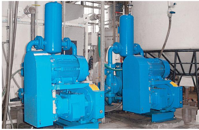
ABEL HMD-G-12-0060 for transfer of contaminated sludge from soil washing process
