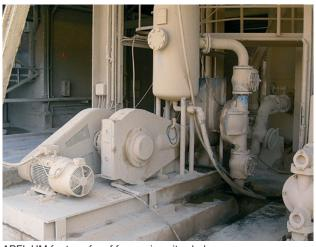
ABEL HM for transfer of ferrous jarosite sludge
