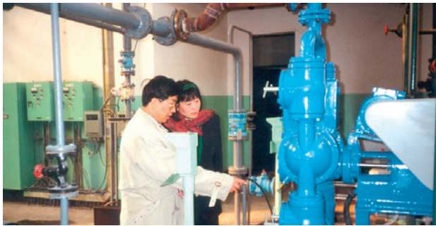
ABEL CM-pump for spray dryer feed
