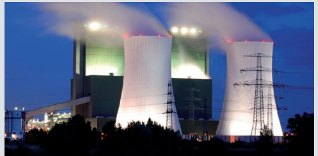
Energy/power plants – flue gas desulphurization
